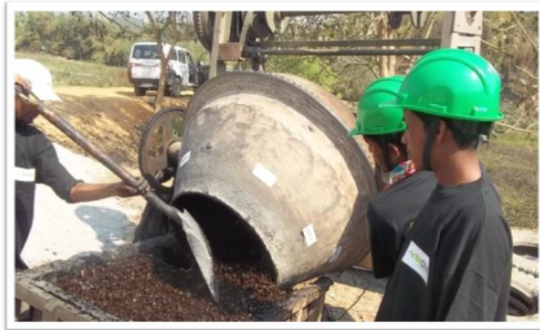
Figure: Coldmix process for road construction
